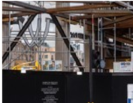
Iconic Whiteleys signs remain in place
