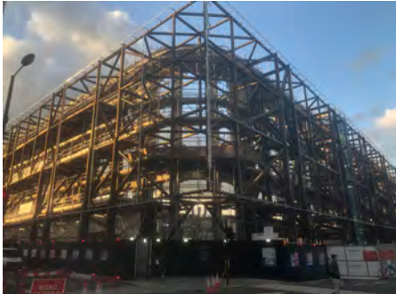
External Facade retention along the Porchester Gardens elevation
