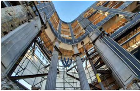
Rear view of the retained historic facade
